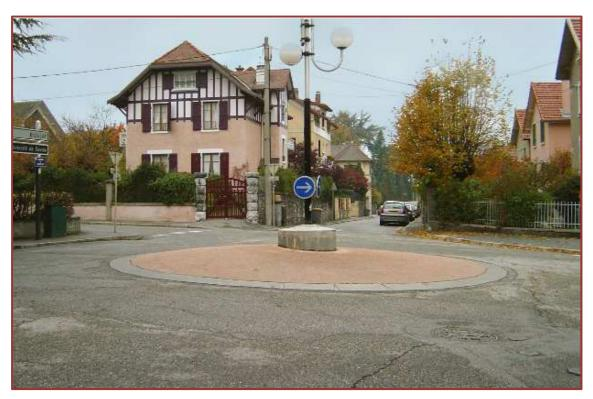
Figure 26: Example of a partially surmountable mini circle
