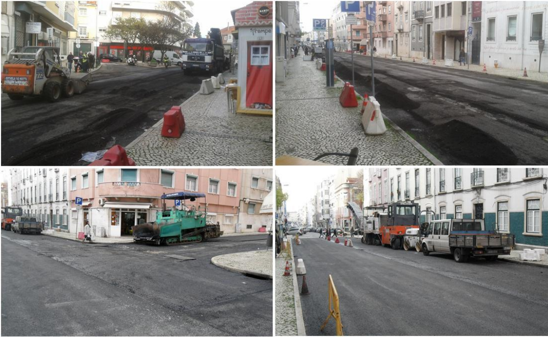
Figure 14 – Pictures of paving works.
