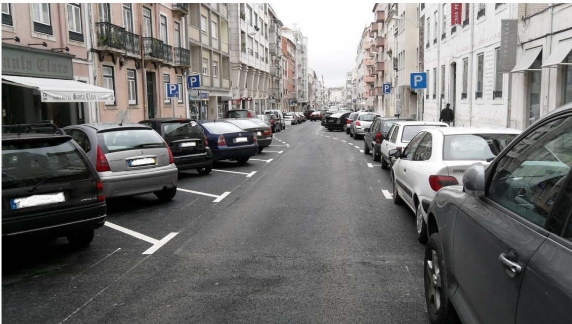
Figure 25 – Picture of the finished works (5).
