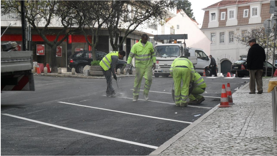
Figure 20 – Picture of the works being carried out (3).
