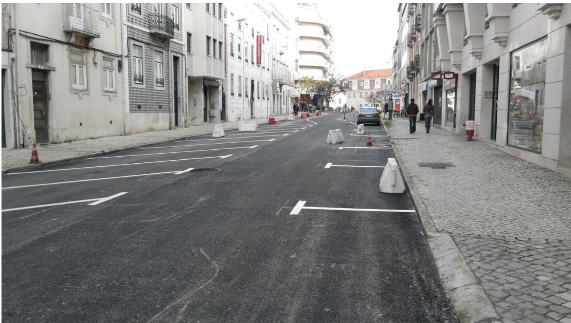
Figure 23 – Picture of the finished works (3).
