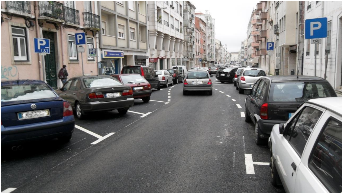
Figure 26 – Picture of the finished works (6).
