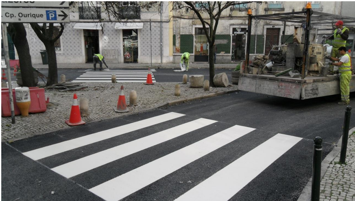
Figure 18 – Picture of the works being carried out (1).
