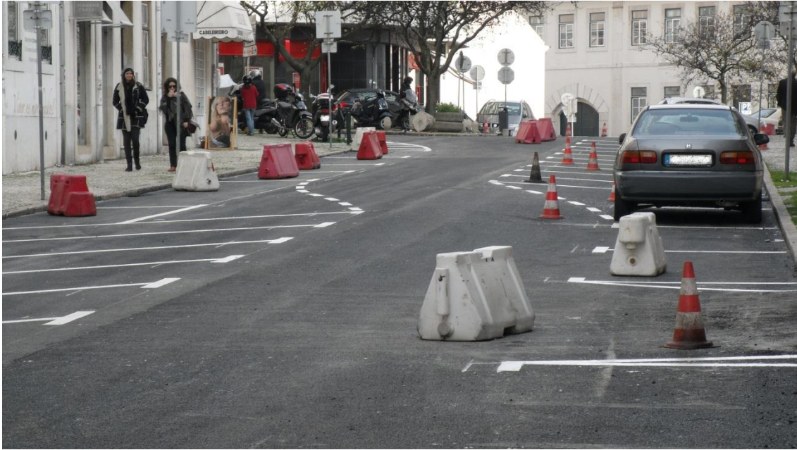
Figure 24 – Picture of the finished works (4).
