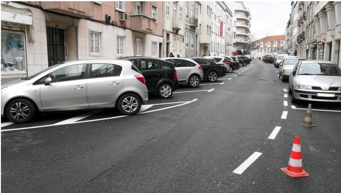
Figure 28 – Picture of the finished works (8).
