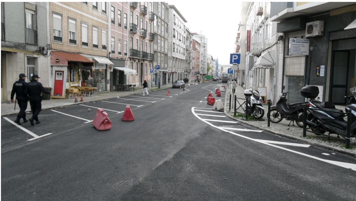
Figure 21 – Picture of the finished works (1).
