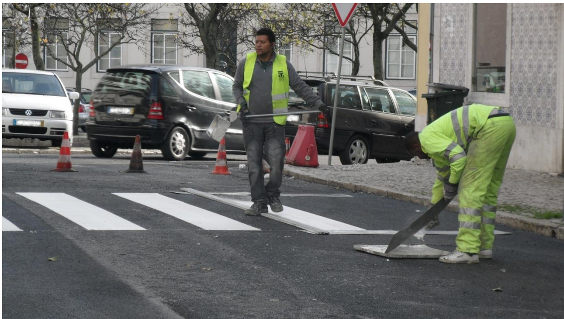
Figure 19 - Picture of the works being carried out (2).
