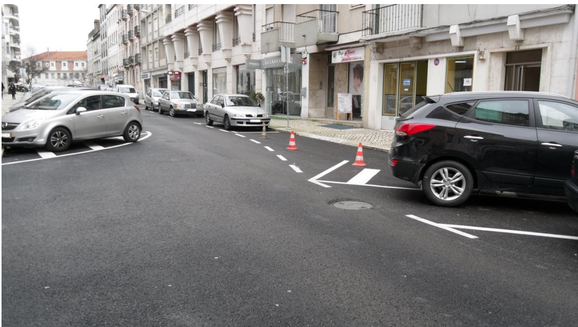
Figure 27 – Picture of the finished works (7).
