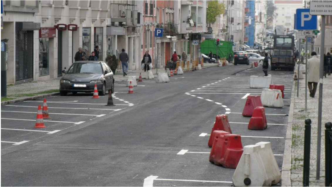
Figure 22 – Picture of the finished works (2).
