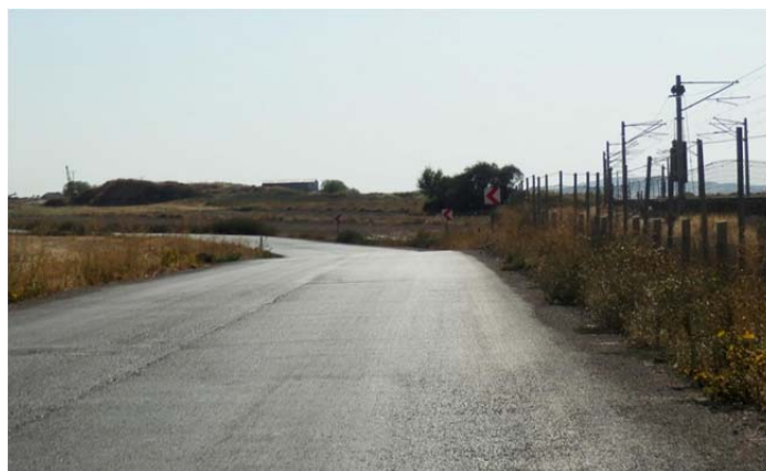
Figure 7. Picture of Project Area Before Implementation
