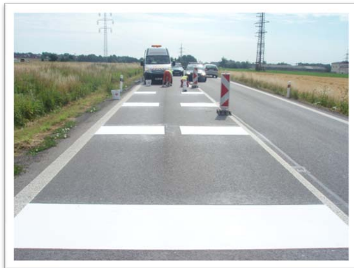
Picture 15: Photo from installation
