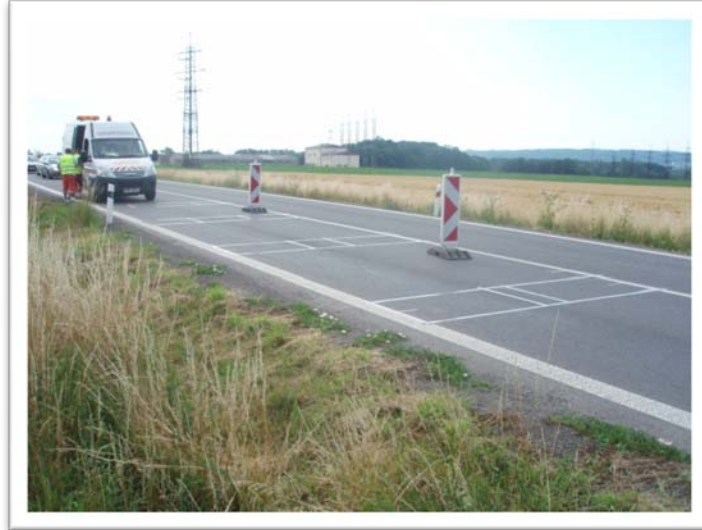
Picture 14: Photo from installation
