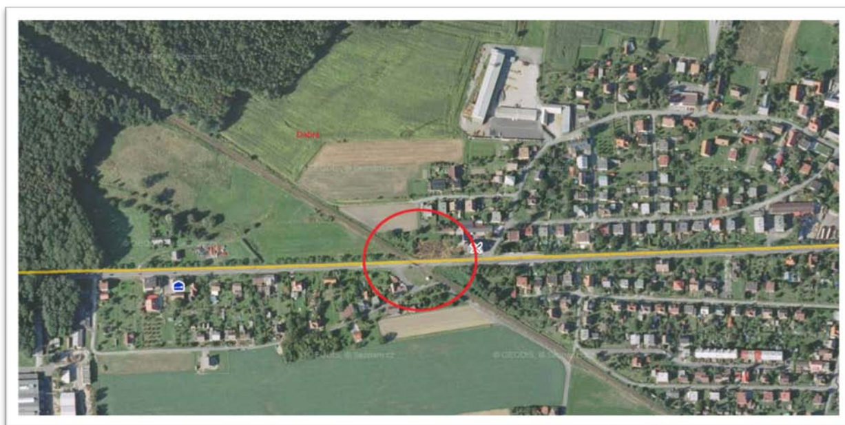
Picture 3: Level crossing in Dobrá
