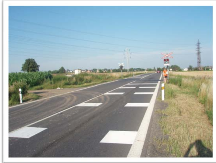
Picture 16: Photo after installation
