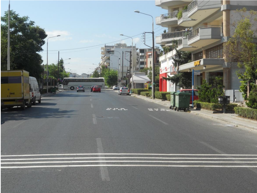
Figure 14: The second set of rumble strips and in the front the label 'BUS STOP'
