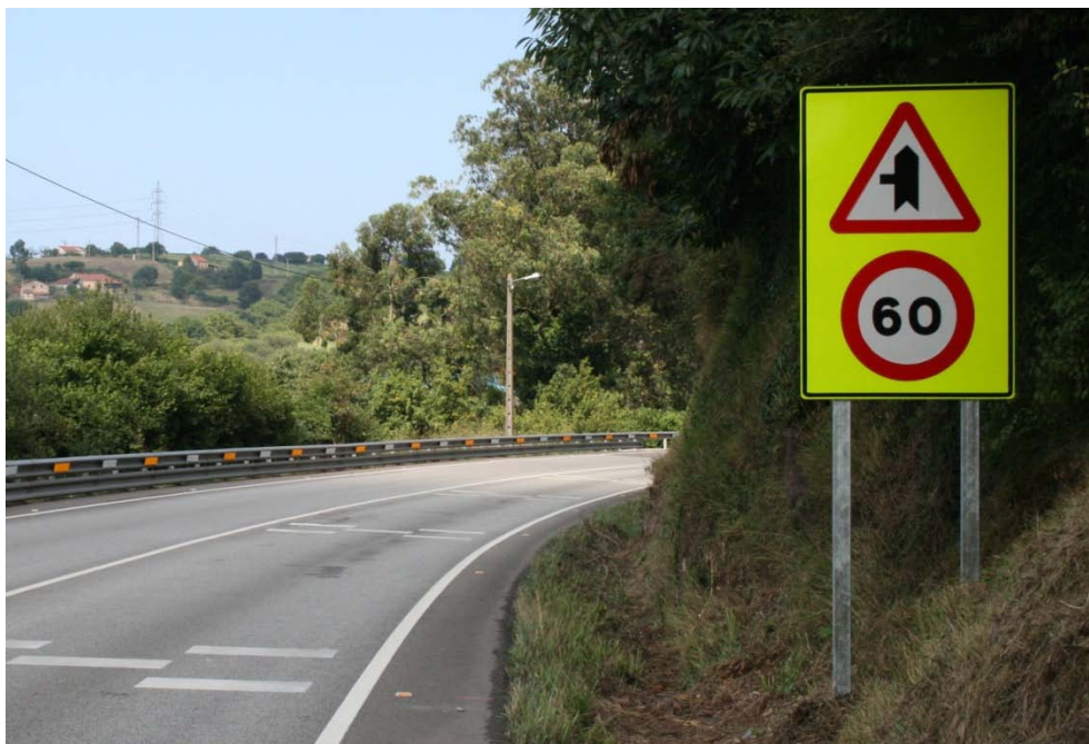
Illustration 40: Panel used to signpost the dangerous crossing and the 60 km/h speed limit.
