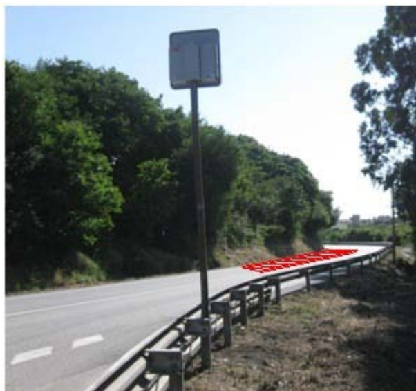
Illustration 41: Stretch in which it is measured the average speed of the vehicles.
