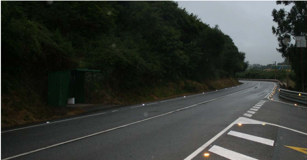
Illustration 37: Looking towards Avilés from the crossing after the 1 st set of actions.
