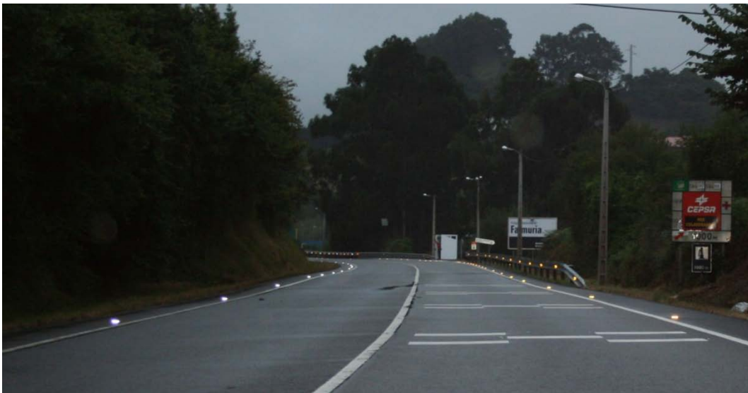
Illustration 38: Looking to the crossing approaching on the way from Gijón to Avilés, after the 1 st set of actions.
