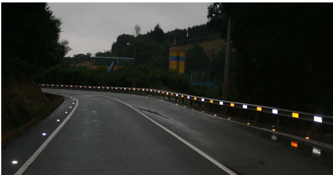
Illustration 36: Delineation of the curve after the actions of the campaign (in the way from Gijón to Avilés).
