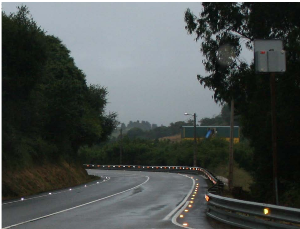
Illustration 39: Detail of the driver feedback sign placed to measure the speed of the vehicles.
