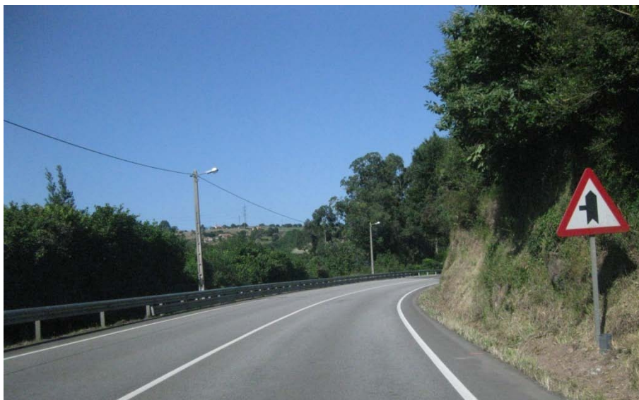
Illustration 28: Aspect of the road after clearing the vegetation from the ditch.
