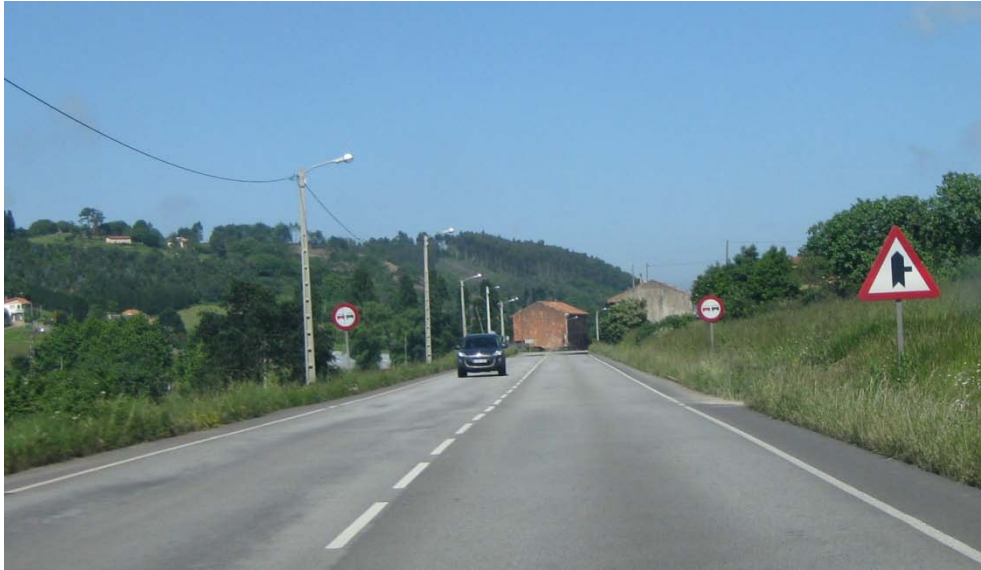
Illustration 57: Signposting of the existence of the crossing in the curve.
