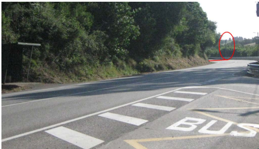
Illustration 17: Visibility distance while trying to incorporate to the AS-19 road from Falmuria Industrial Park.
