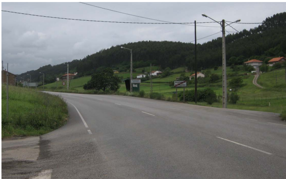
Illustration 56: View from the crossing, on the way from Avilés, visibility is too small.
