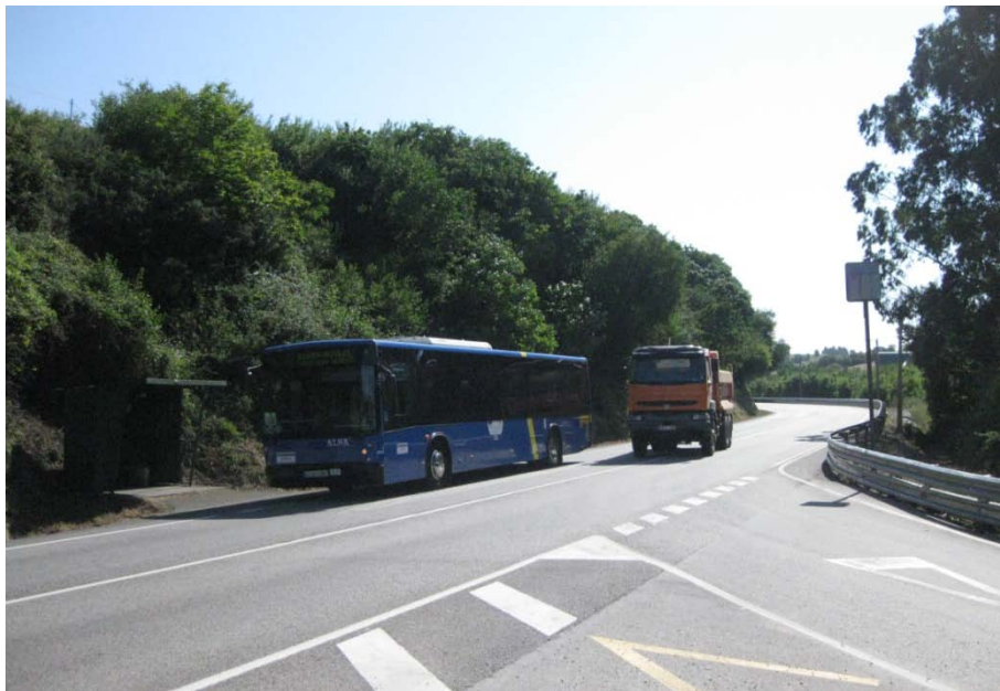
Illustration 33: Location of the radar and detail of a dangerous situation during the bus stop.
