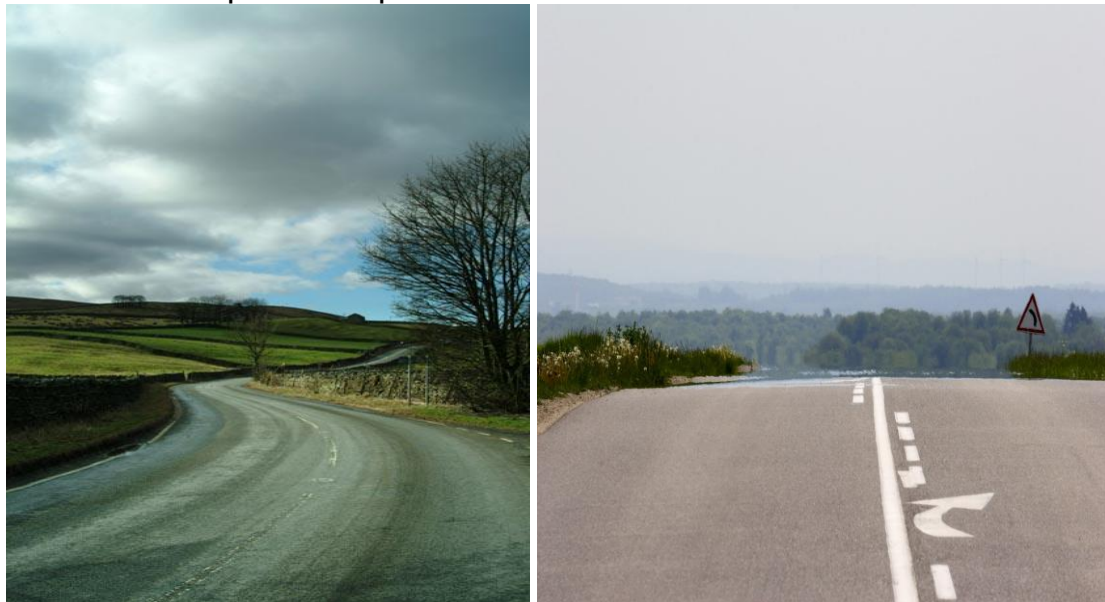
Single carriageway with poor markings and single carriageway with poor visibility
