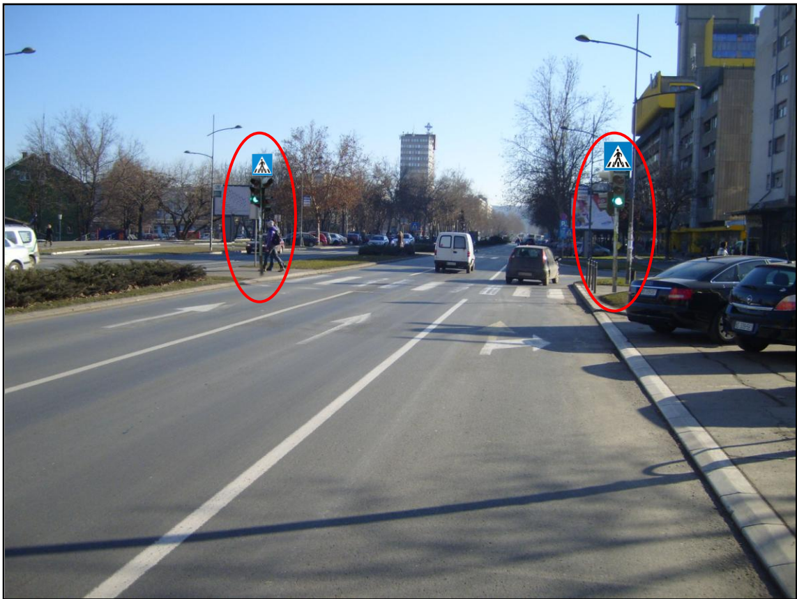
THE HIGH RISK SITE AFTER TREATMENT
