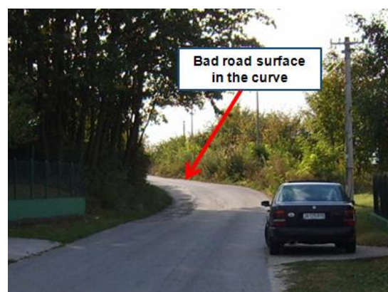
Photos 4. and 5. Black spot C problems - holes on the road surface provoke dangerous maneuvers
