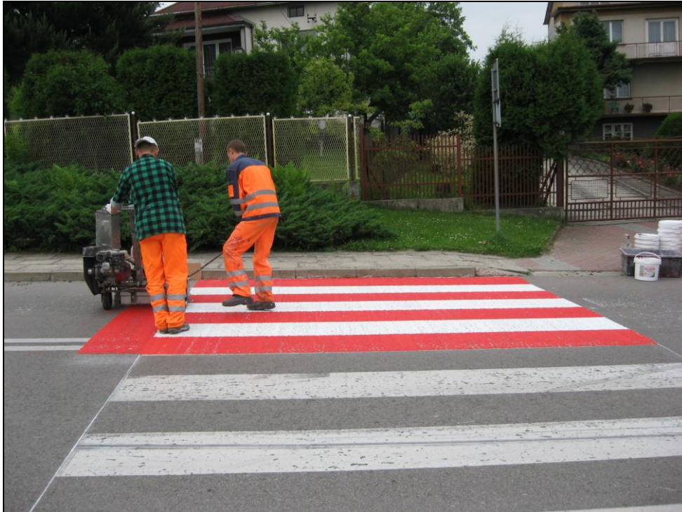
Pictures 4.1.,4.2. Making of new pedestrian crossing on a red surface.
