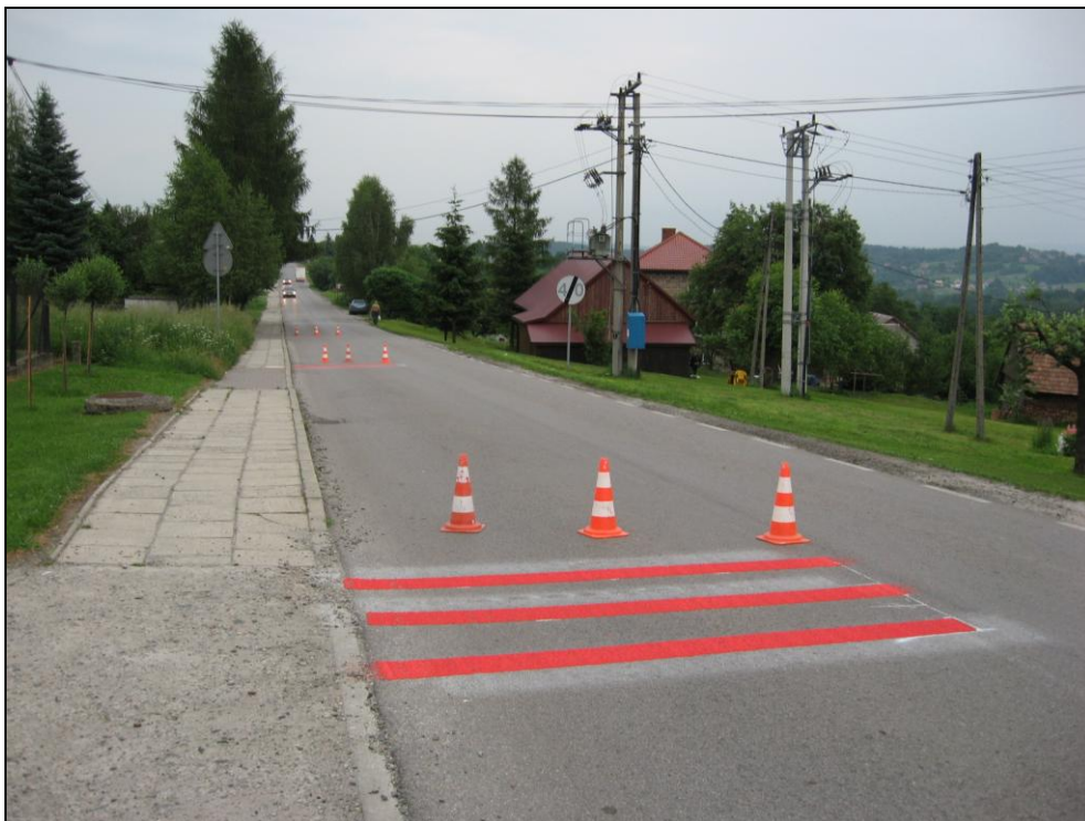
Picture 4.3. Acoustic lanes before pedestrian crossing.
