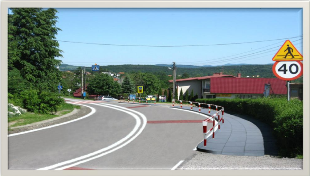
Pictures 2.3.-2.4. High risk site after changes
