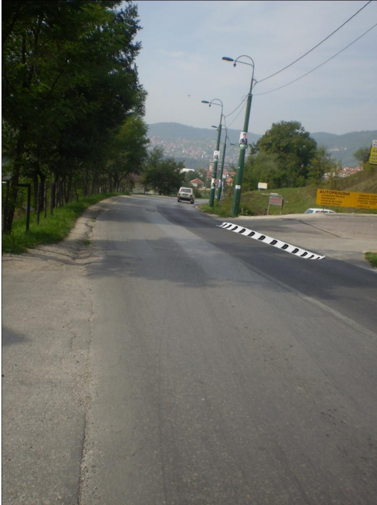
Picture 9.: Proposal to treat high risk site: Set the grid and provide the best possible drainage
