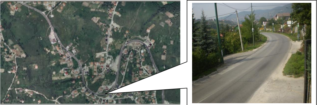
Picture 5.: Problem: Curves, lack of visibility, lack of traffic signs
