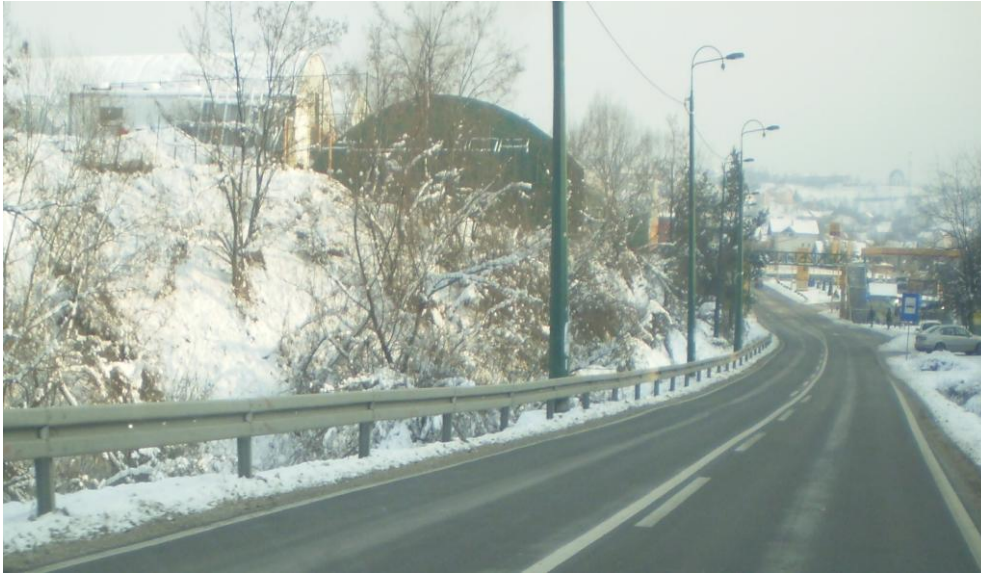
Picture14.: Installation of protective crash barriers
