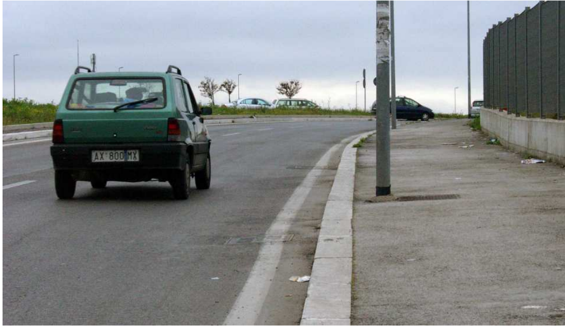
10 - The view of a motorist at 83 meters from the intersection at grade.
