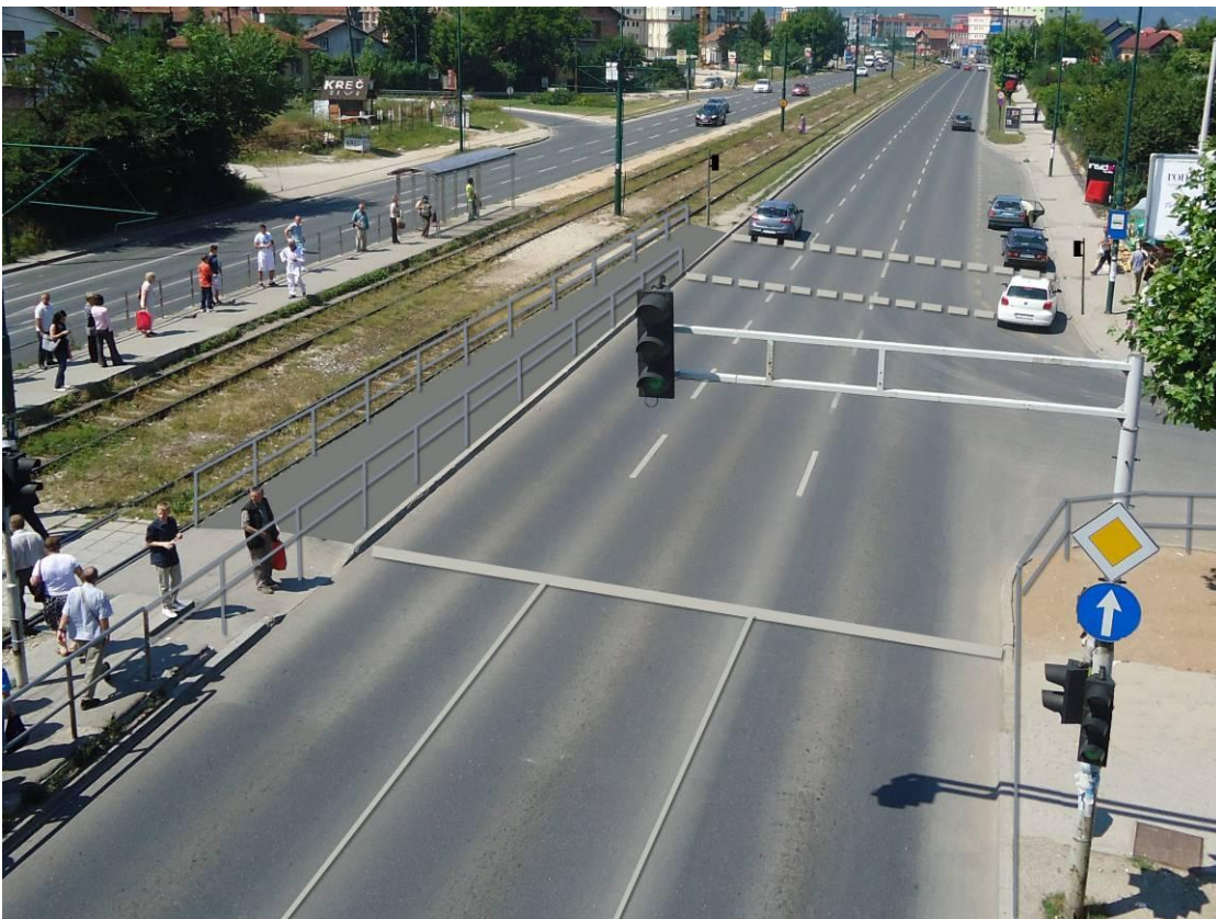
Figure 15: High – risk site before and after (computer simulation) implementation of first and second set of proposed measures
