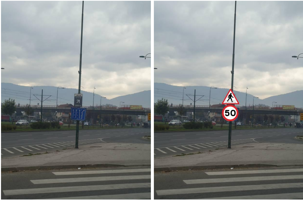
Figure 8: Before and after (computer simulation) the second set of measures – ‘Pedestrian crossing’ and speed limit signs 150 meters in front of the crossing
