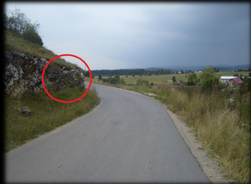
Figure 6. Insufficient visibility caused by rock
