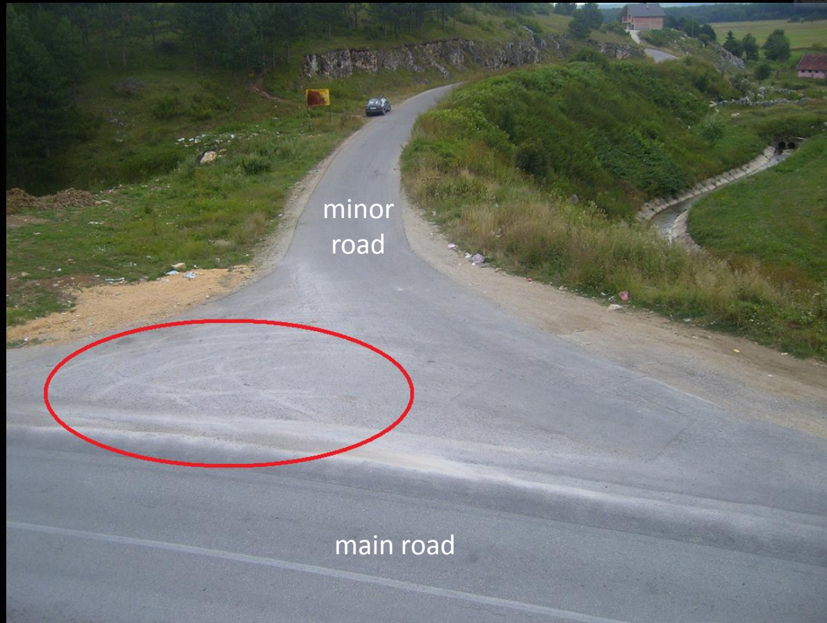
Figure 4. Intersection of roads
