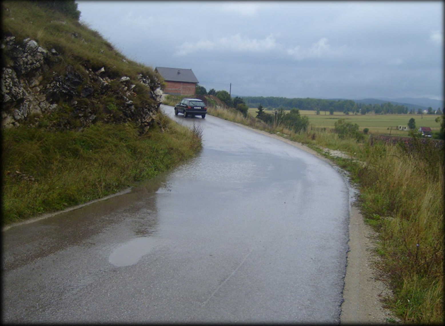
Figure 8. Rainwater on the carriageway
