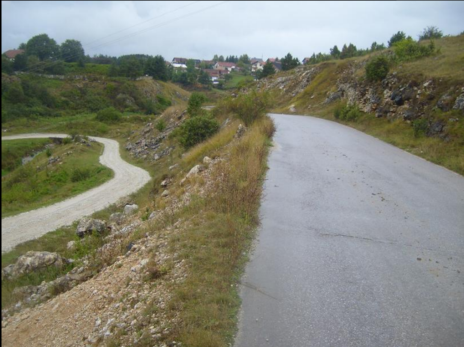
Figure 12. There is no protective crash barriers for vehicles
