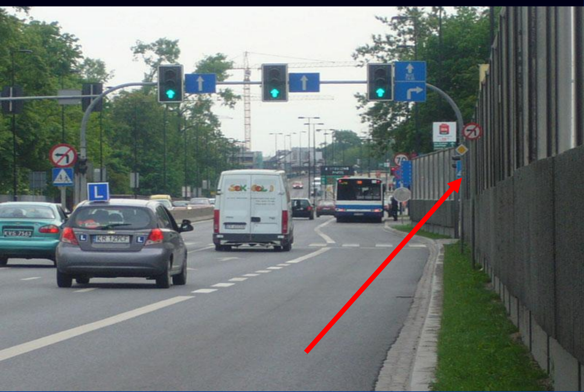
Pedestrian crossing sign is not well seen, some signs are too small
